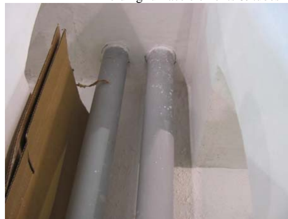
Holding furnace elements & tubes
